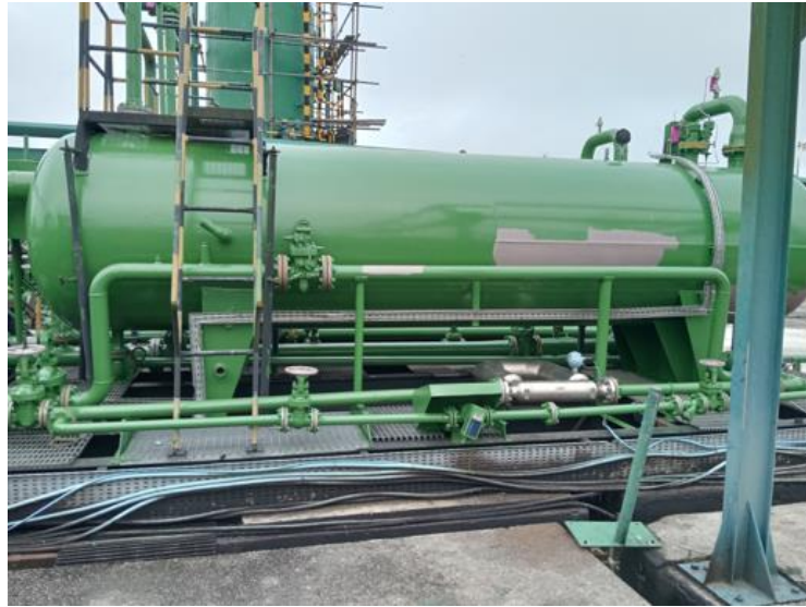
Fig 5: A typical test separator (2-phase)
