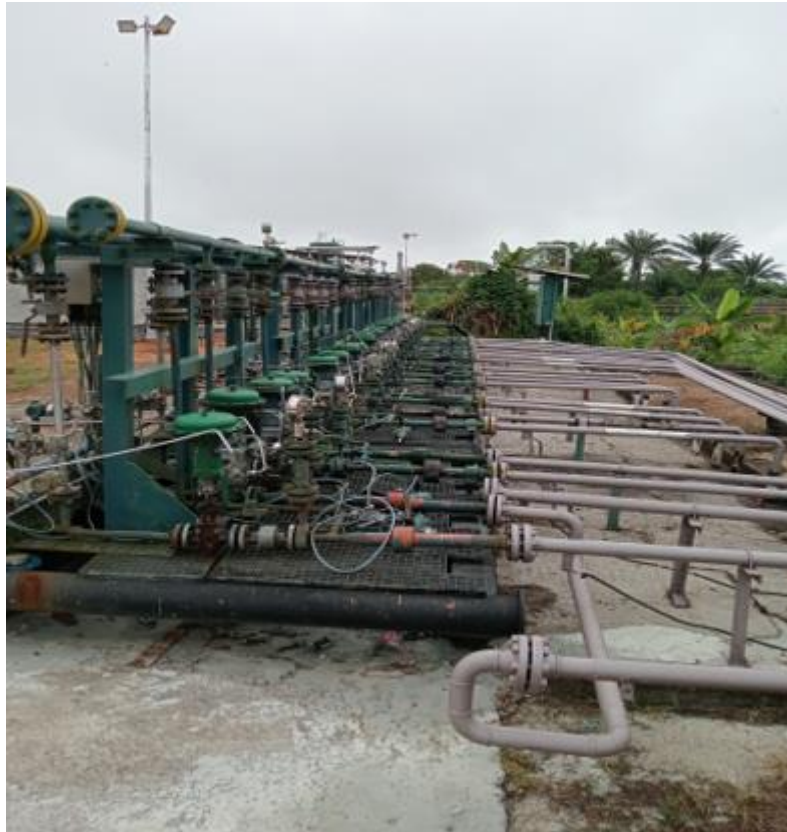
Figure 2: A typical GDM assembly
